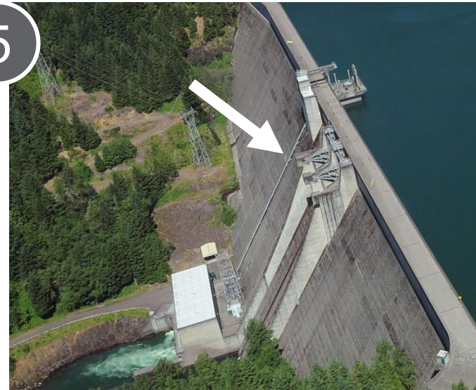
Bypass pipe passage Bypass pipe passage
