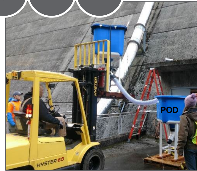
Forklift/ Flex hose/ Pod holding Enter FSS/ Chute passage/ Pod holding
