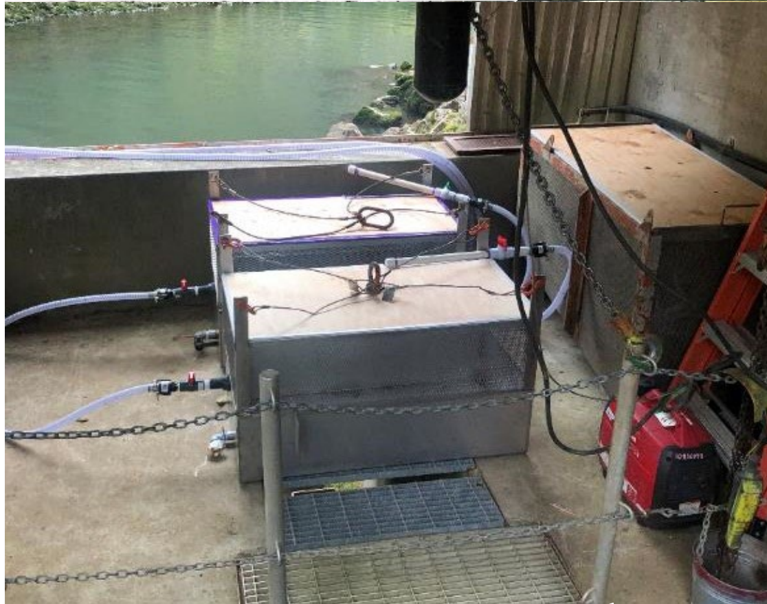
Bypass Pipe Fish Collector
